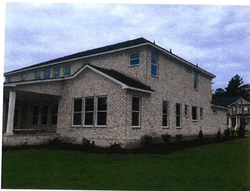
Photo Two Caption LEFT VIEW 6/26/2018
