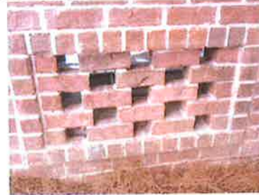
TYPICAL GARAGE DOOR FLOOD VENT 5/09/2012
