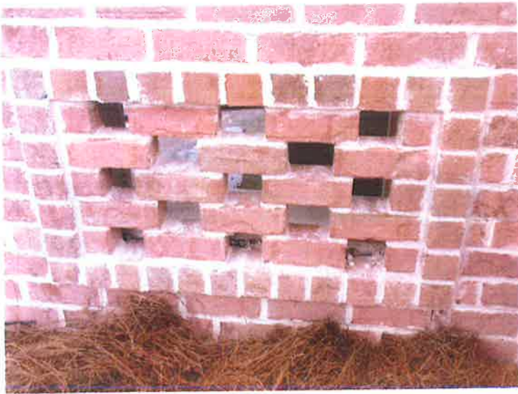
GARAGE DOOR WITH 2 FLOOD VENTS 5/09/2012
