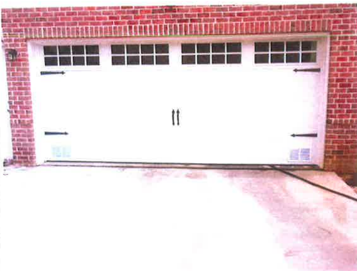
GARAGE DOOR WITH 2 FLOOD VENTS 5/09/2012
