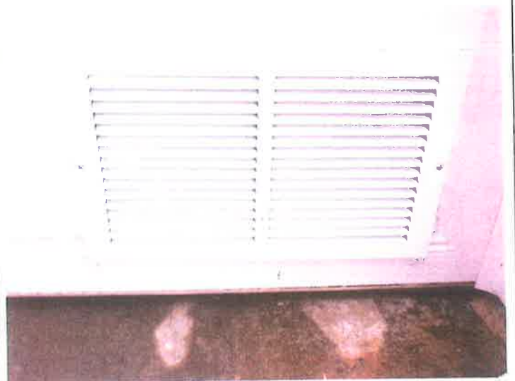
TYPICAL GARAGE DOOR FLOOD VENT 5/09/2012
