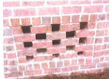
GARAGE WALL FLOOD OPENING (3 OF 3)
