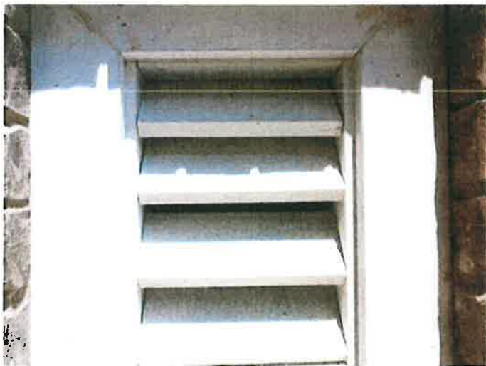
(TYPICAL) FLOOD VENT IN GARAGE WALL 4/01/2013
