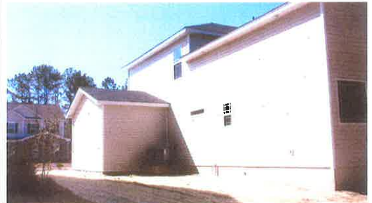
RIGHT SIDE VIEW/CONDENSING UNIT 02/24/2011
