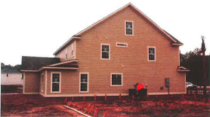
LEFT SIDE VIEW/CONDENSING UNIT 1/25/2011
