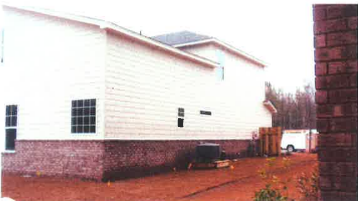
LEFT SIDE VIEW/CONDENSING UNIT 2/10/2010
