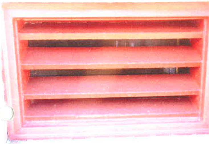
INTERIOR VIEW OF TYPICAL FLOOD OPENING IN FRONT ENCLOSURE(GARAGE) WALL 11/19/2011
