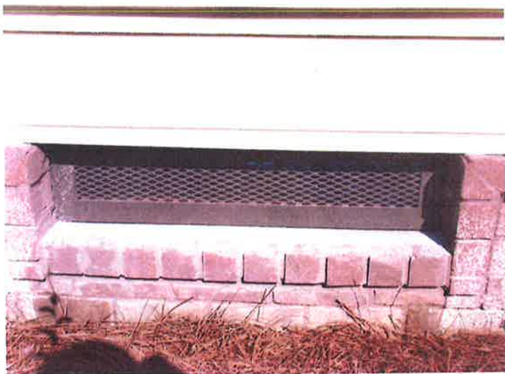
WIRE MESH VENT IN EXTERIOR GARAGE WALL 5/24/2012
