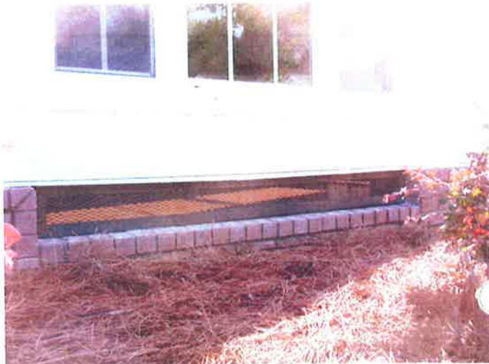
WIRE MESH VENT IN EXTERIOR GARAGE WALL 5/24/2012
