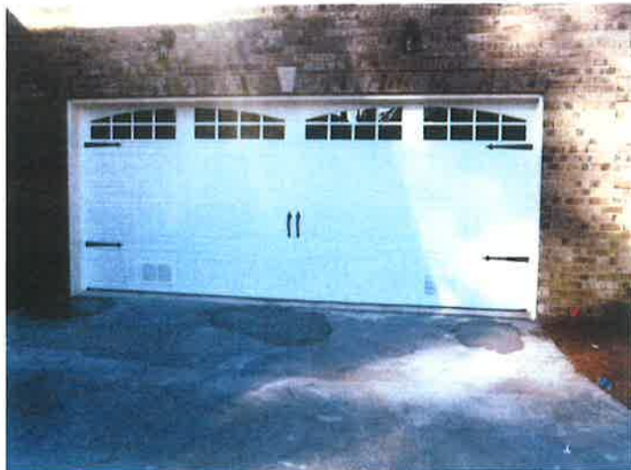
TYPICAL FLOOD OPENING IN ENCLOSURES(GARAGES)
