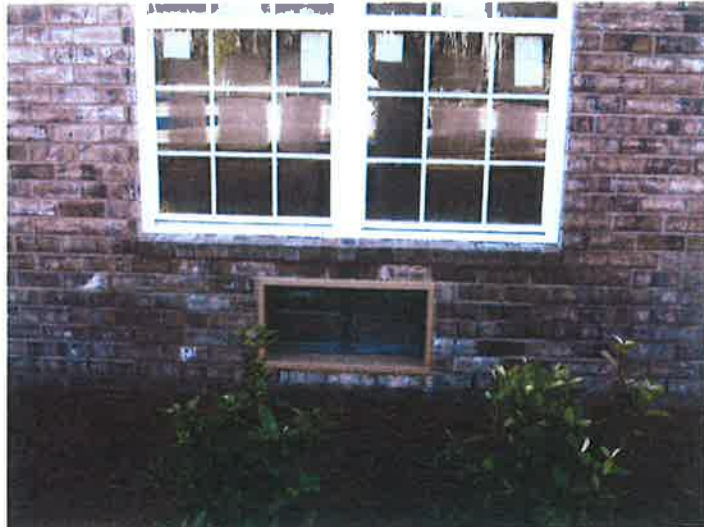
TYPICAL FLOOD OPENING IN ENCLOSURES(GARAGES)
