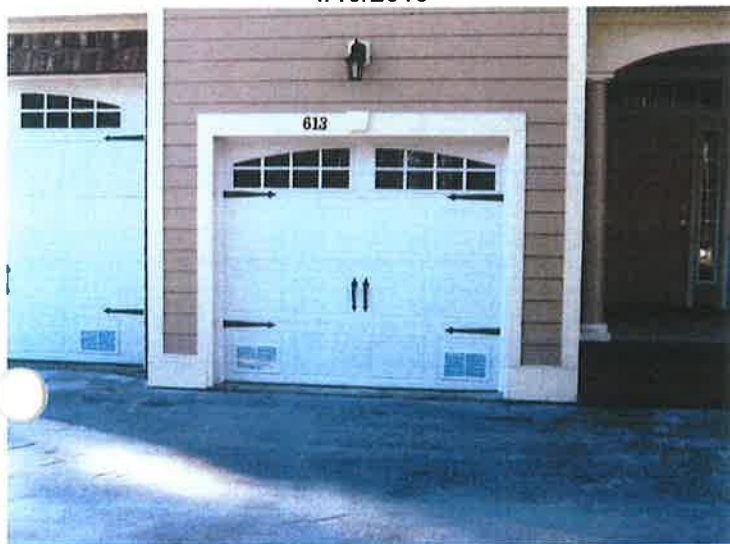
TYPICAL FLOOD OPENING IN ENCLOSURES(GARAGES)
