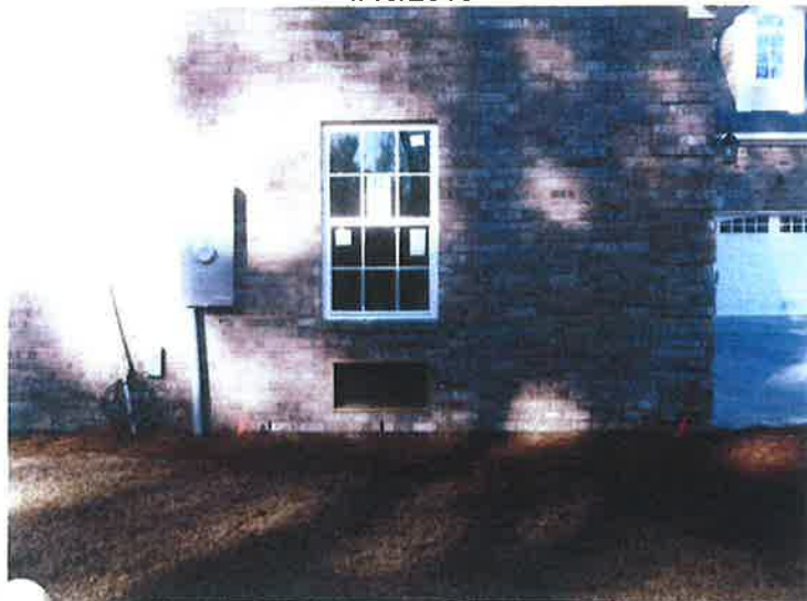
TYPICAL FLOOD OPENING IN ENCLOSURES(GARAGES)
