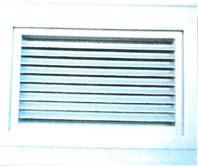
(TYPICAL) FLOOD SOLUTIONS LLC FLOOD VENT IN GARAGE DOOR 2/25/2013
